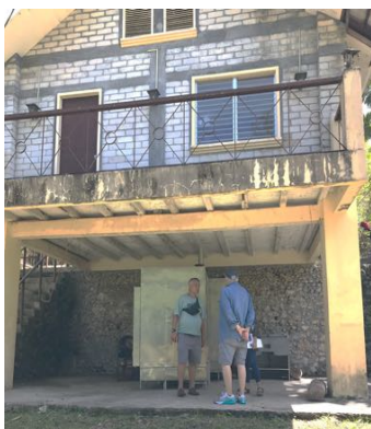
Building renovated for micro-processing plant
